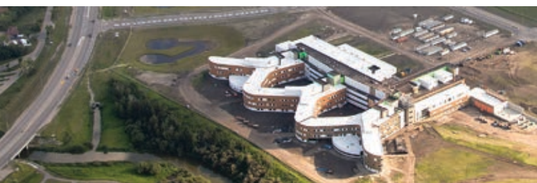
Construction of the new Grande Prairie Regional Hospital
